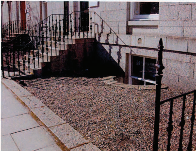
Photo 2 Albert St – Typical absence of Railings and lack of Landscaping:
