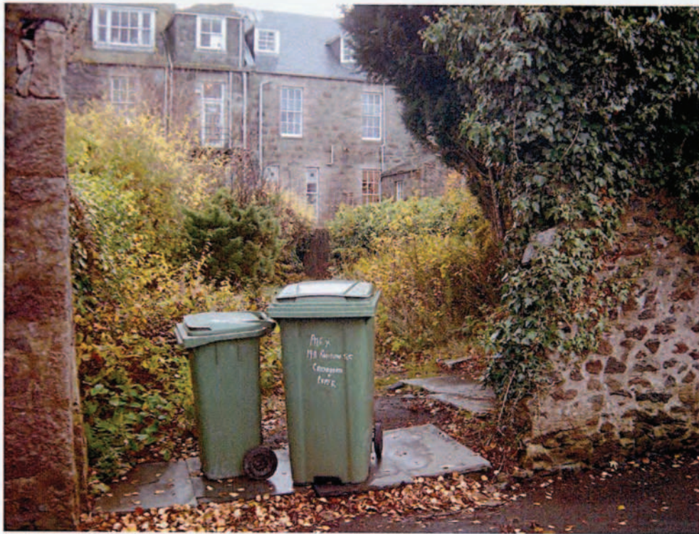
Photo 5 'Breached' Victorian wall To create car park – Rubislaw Tce lane.
