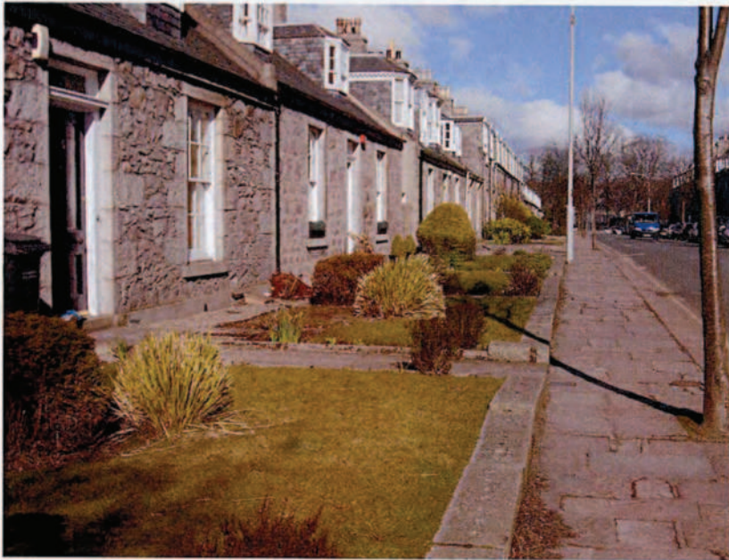
Photo 1 Victoria St - Showing absence of original Cast-iron Railings:-
